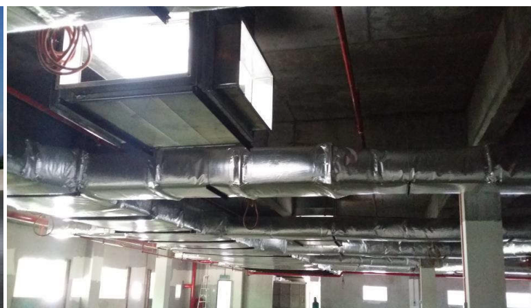
HVAC, Exhaust and Ventilation Ductwork were installed.
