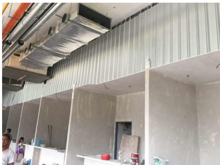
HVAC, Exhaust and Ventilation Ductwork were installed.
