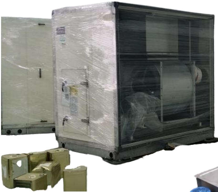
Air Handling Unit (AHU)
