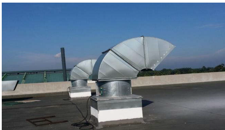
HVAC, Exhaust and Ventilation Ductwork were installed.
